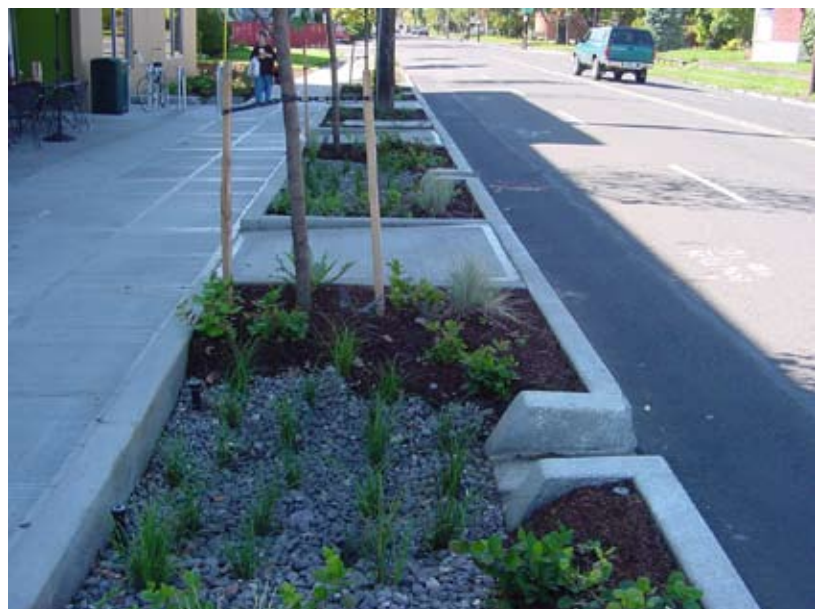
Periodic curb cuts allow for streetside infiltration of stormwater, reducing the amount of runoff that enters storm sewers.
