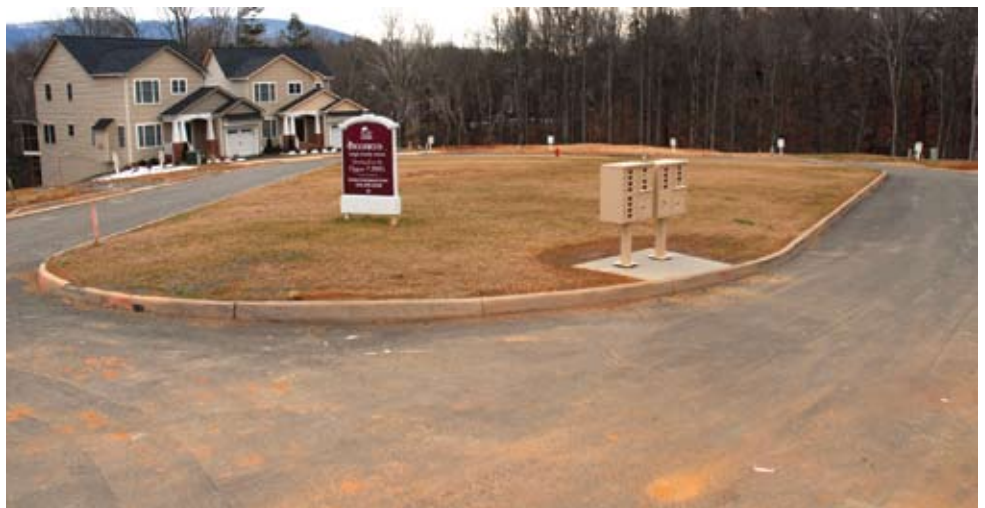
This is a good example of a landscaped island in the middle of a cul-de-sac, located in the new Brookwood development currently under construction on Raymond Avenue in Charlottesville. Additional stormwater benefits could be provided if it were designed so that runoff from the street drained into it.
